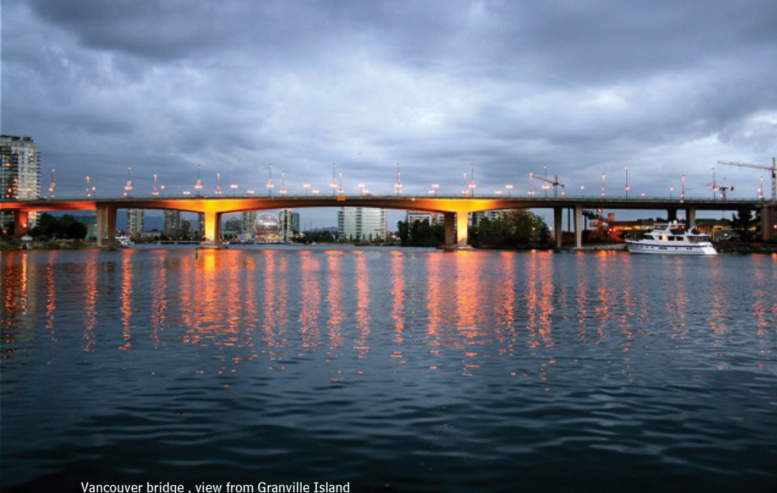
Vancouver bridge , view from Granville Island
